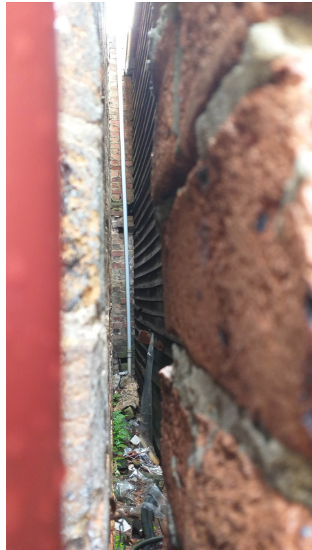
Figure 97: View between Griffin Theatre (left) and 12 Nimrod Street showing timber weatherboard cladding on north facade of the terrace house.
