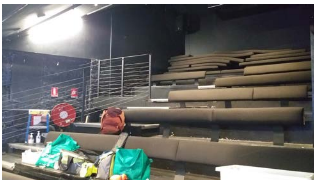
Figure 130: Tiered theatre seating. Source: TZG Architects, 2022.
