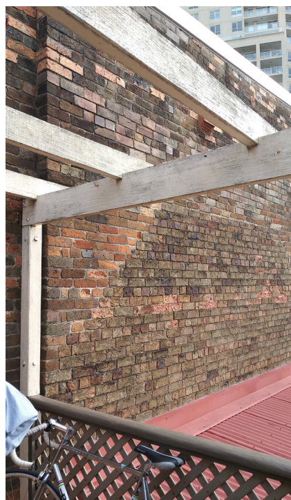
Figure 157: View of brick repairs to external wall of SBW Stables Theatre. Roof over kitchen visible.
