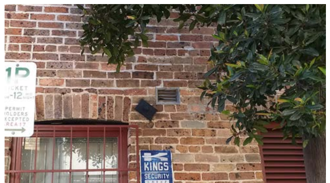
Figure 110: Metal element possibly associated with original stable doors (now removed) on main facade.
