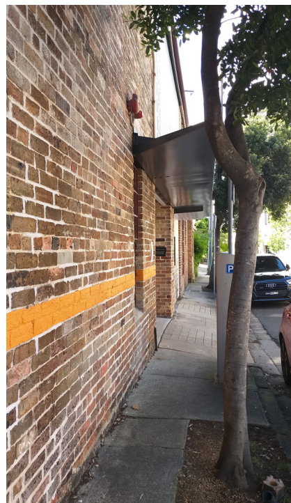
Figure 104: View along Nimrod Street of steel awning above the main entrance to the theatre.
