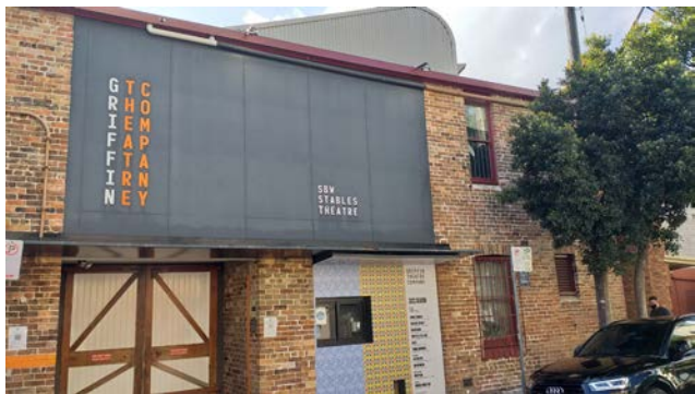
Figure 93: View of main facade along Nimrod Street with small verandah roof the 12 Nimrod Street visible on the right.
