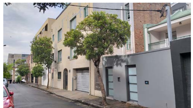
Figure 89: View of properties located opposite the subject site. Source: TZG Architects, 2022.
