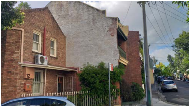
Figure 84: View of house at 12 Nimrod Street at the corner of Nimrod and Caldwell Street. The house forms the southern extent of the subject site. Source: TZG Architects, 2022.
