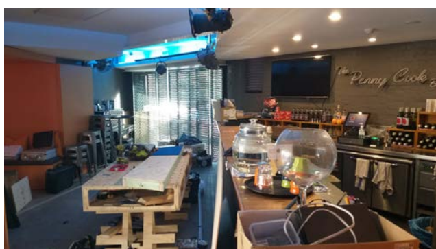
Figure 116: Main foyer, lobby and bar area currently used as a workshop. Source: TZG Architects, 2022.
